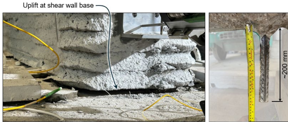
Figure 11. Observed failure mode in wall S2.
